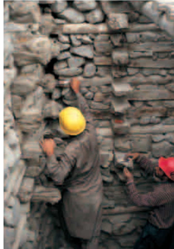
Monitoring structural movements during restoration works.
