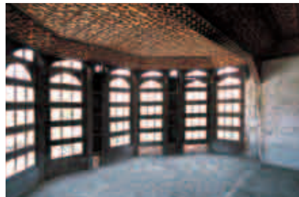
Front facade of Khaplu Palace (above) and interior of the projecting room on the upper floor.
