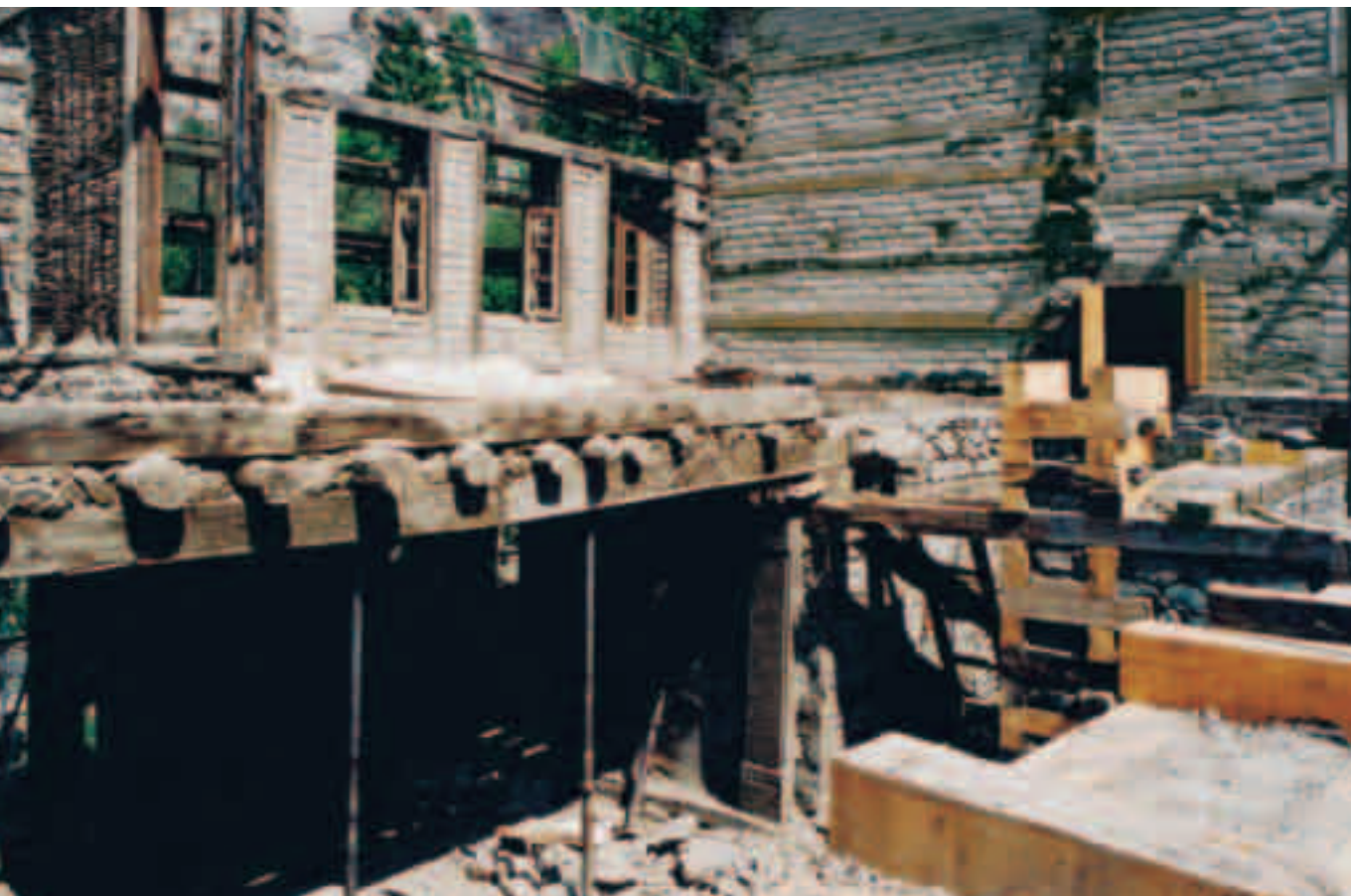
Below: Module I reception hall after removal of the infill wall and before extending the hall to its original size.
