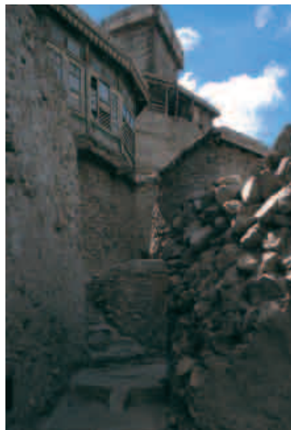
The rehabilitated main spine of Altit village leading up to the Fort, after introducing new sanitation lines and stone pavements.
