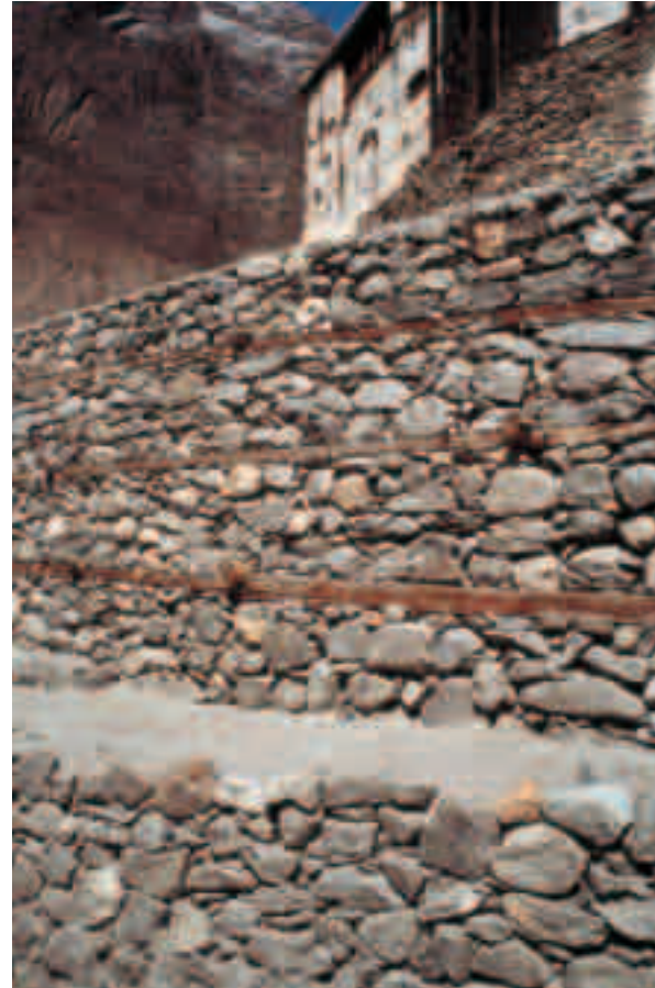
Restored retaining walls at the foot of the fort.
