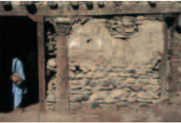
Above: The central column of the former reception hall "buried" in later infill construction.
