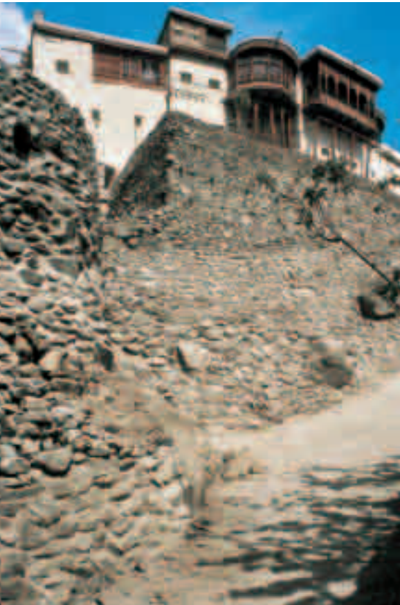
View of the western front side of the restored Baltit Fort, from the steep stone-paved walk-way leading up from the village. The windows and balconies of the early-20th century additions are clearly seen. (For interior views see pages 23 and 29.)
