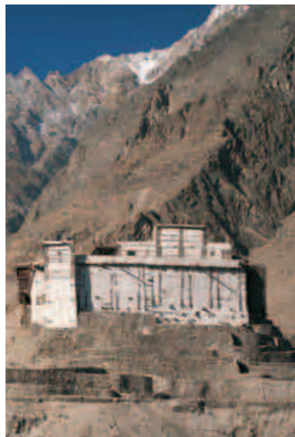
Baltit Fort from the north (back) side, facing the ravine, after restoration was completed.
