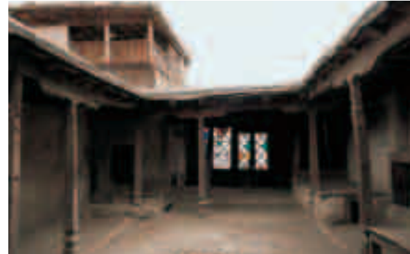
Above: The Queen's ("Rani's") summer courtyard on the second upper floor. Below: A detail of the restored western bay window.
