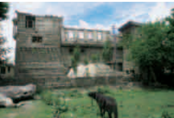
Above: Entrance to the Shigar Fort complex (unrestored) with the “Old House” on the left.
