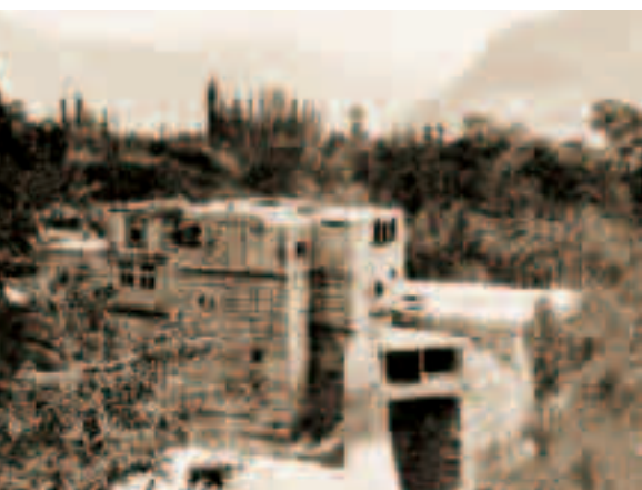
An old photograph of Shigar Fort (around 1900), showing upper floors on the north-eastern corner which have since collapsed.
