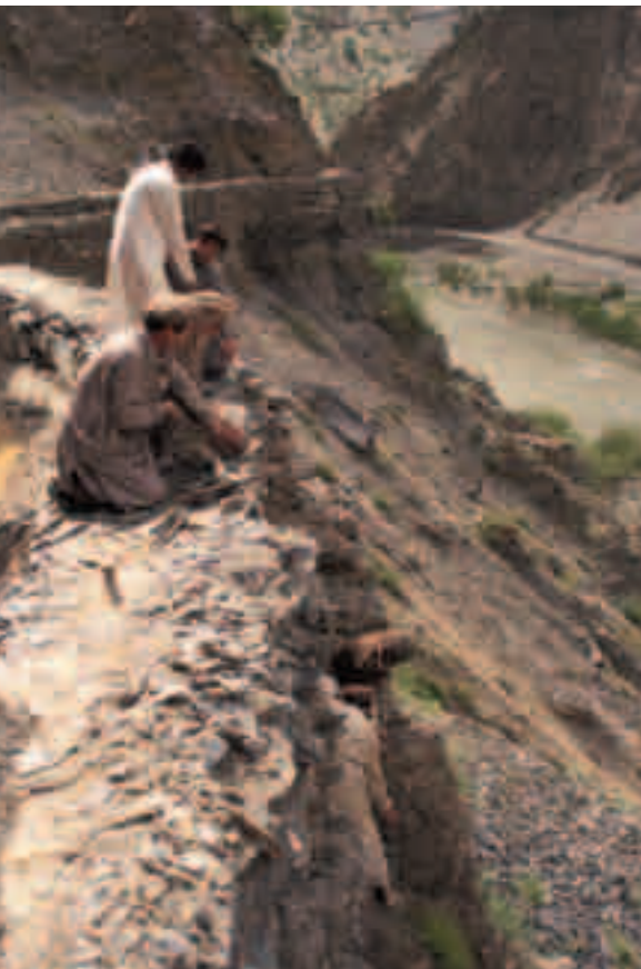
Villagers reinforcing the walls of an irrigation channel, which parallels the river below.
