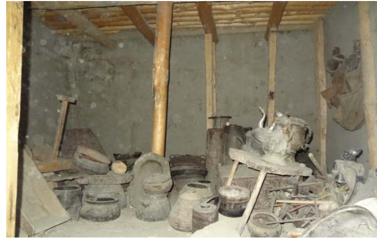
One of the rooms at Ground Floor presently being used as a store
