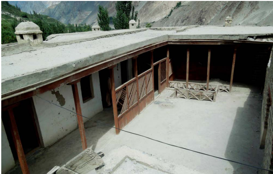
View of the First Floor having rooms around the terrace
