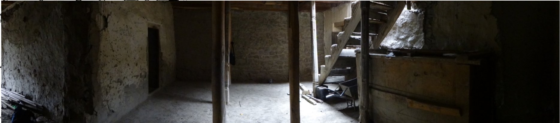
Interior view of the Ground Floor
